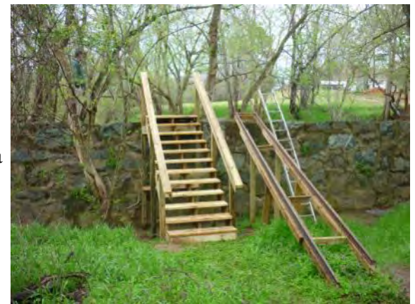
Newly Constructed Portage Steps over Puryear Dam
