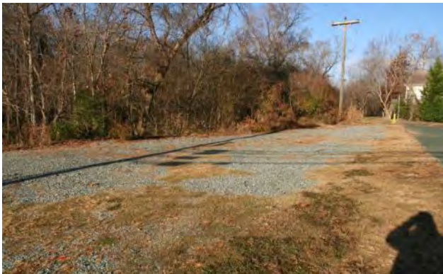
Saxapahaw Mill Race Paddle Access before the renovations
